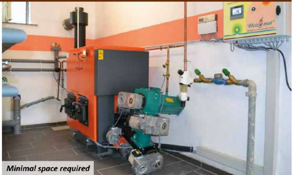
Automatic combustion chamber deashing
